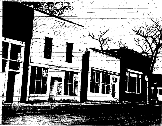
GOING DOWN: One of the oldest buildings in Allen (second from left) is now being torn down to make room for future expansion by the Allen bank.
